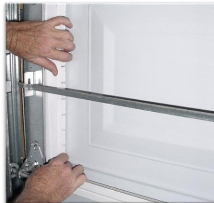
Step 4. Insert the excess insulation behind the vertical rails
