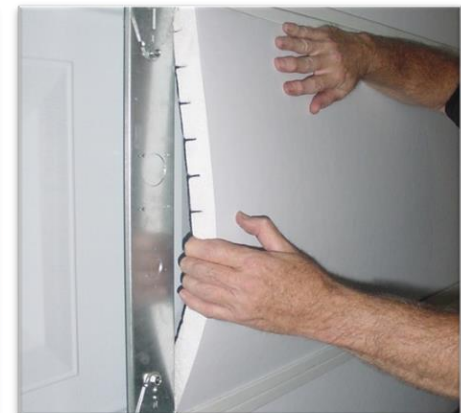
Step 5. Insert the insulation sheet between the horizontal rails
