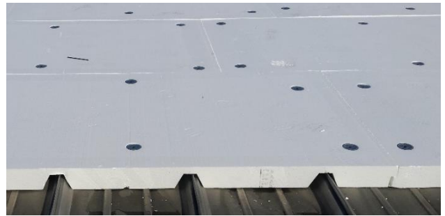
Laminated Flute Fill Combo Board with an FR facer (above) and a polyester facer (below), over which a PVC roofing membrane was directly installed.
