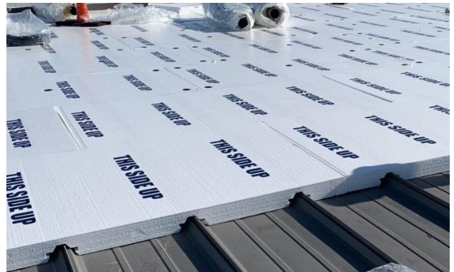
Laminated Flute Fill Combo Board with an FR facer (above) and a polyester facer (below), over which a PVC roofing membrane was directly installed.
